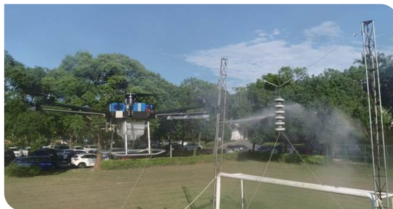
Drone-Based Insulator Cleaning Operation
